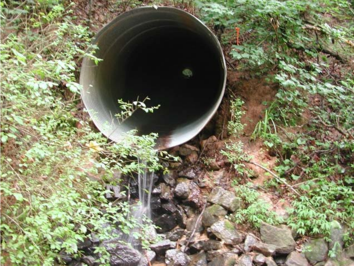
Figure 9: Stormwater outfall. Photo credit: Jeremy Pike.
