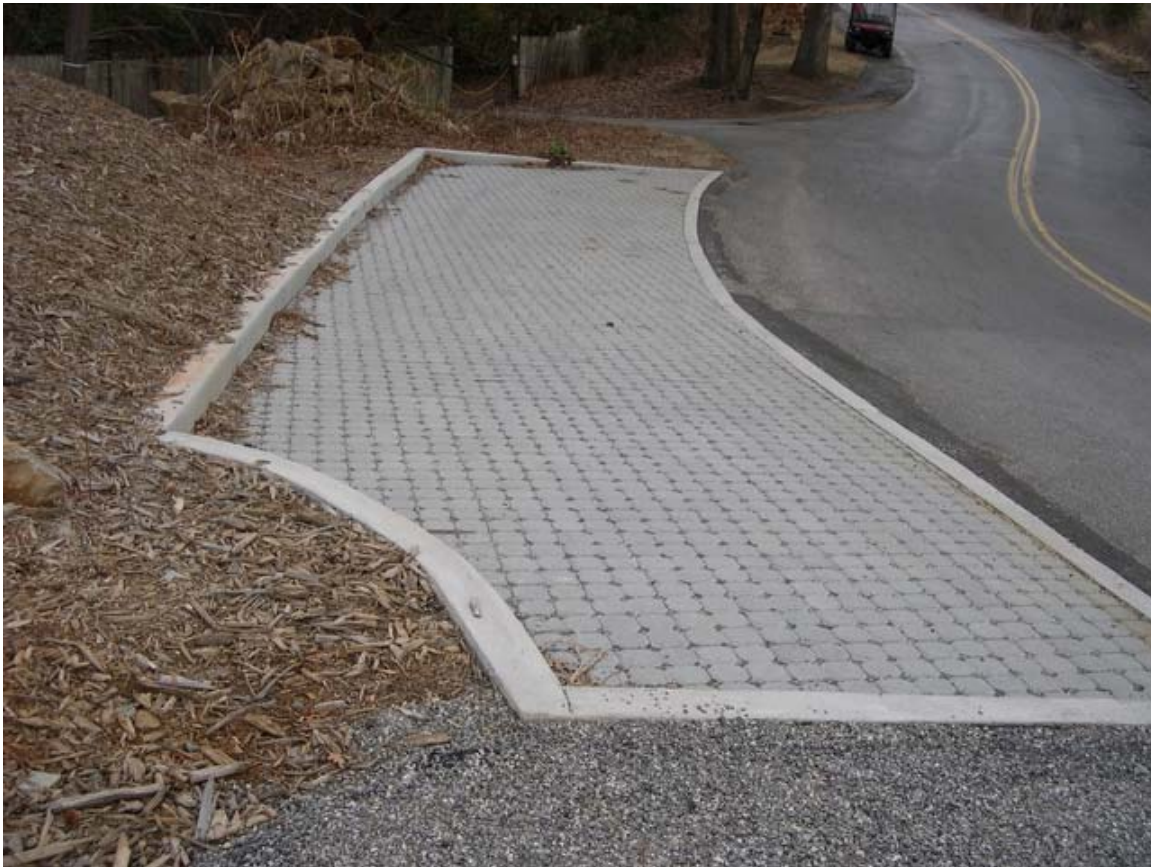
Figure 14: Permeable Paving for Bus Parking.
